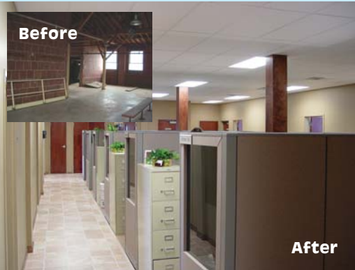
Circa 1940's change houses transformed into modern offices for Esterline Defense Group at Milan Commercial Complex, TN
